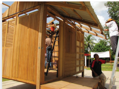
HOOR 3: Finalising fixing of roof panels
