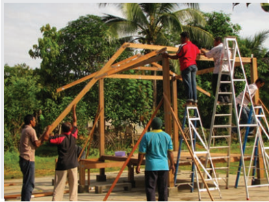
HOOR 1: Main structural components were assembled
