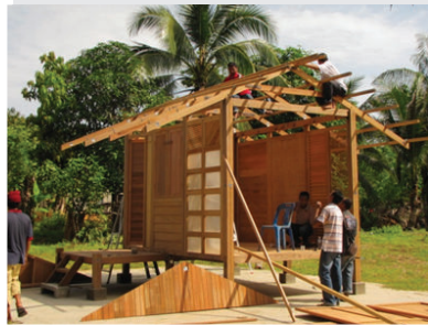
HOOR 2: Assembling wall module completed within the second hour
