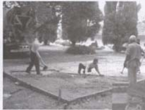
◀ Figure 4. Mortarless construction and self-aligned features of the Putra Block™
